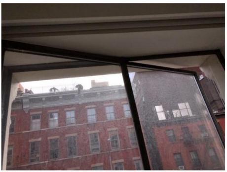
Steel Windows with Minimal Frame and No Brick Mold
