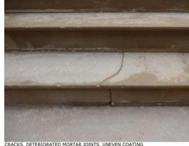
CRACKS, DETERIORATED MORTAR JOINTS, UNEVEN COATING
